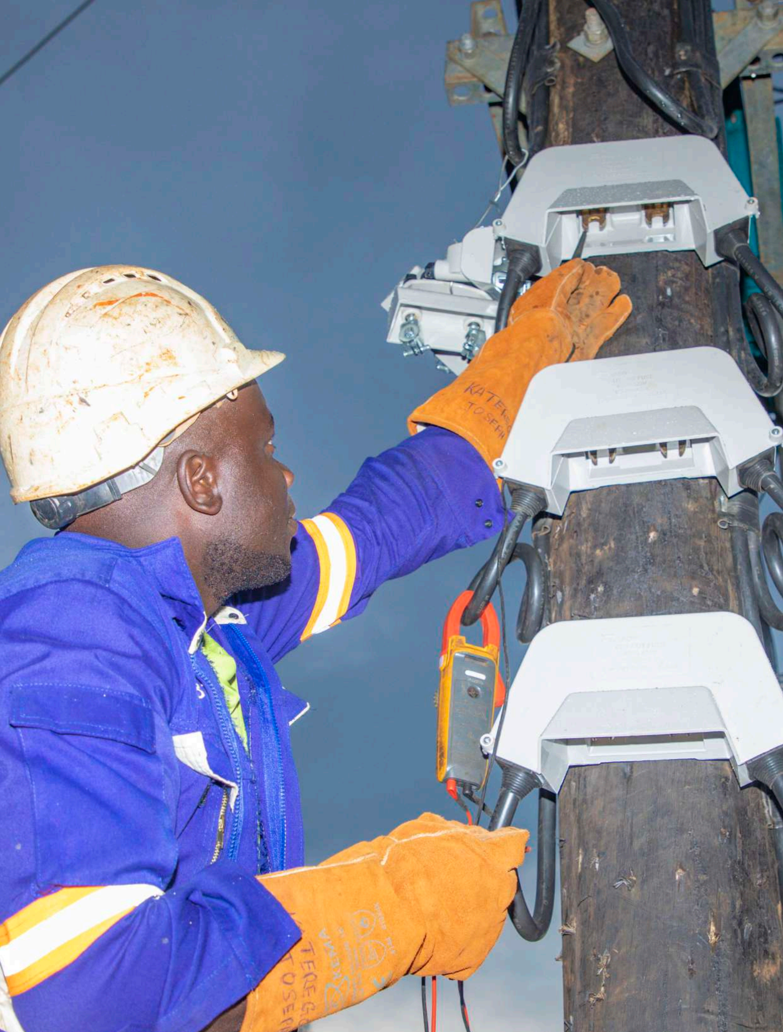
UEDCL Technician running pre-tests following installation of a new transformer
