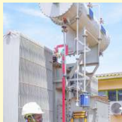
Distribution Concession Monitoring
